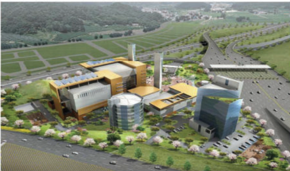
Cogeneration Plant Hot Water / 210RT 4units, 180RT 3units
