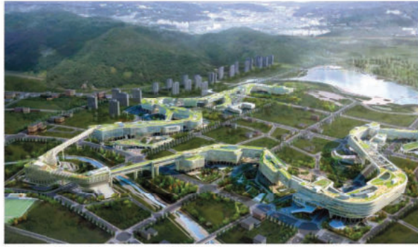
Sejong City Government Office Hot Water / 600RT 8units
