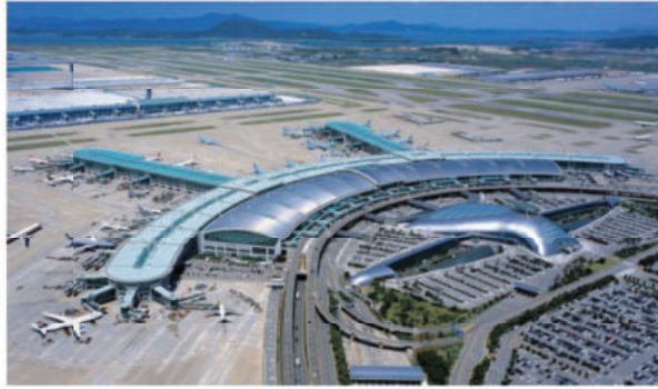
Incheon Airport Hot Water / 975RT 8units
