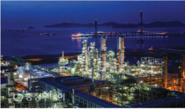
Lotte Chemical Industry Hot Water / 1300RT 3units, 975RT 1unit
