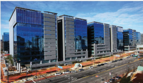
Korea Venture Town Hot Water / 340RT 6units, 300RT 4units
